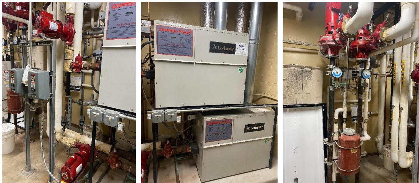
**Description:** The Community Center was constructed in 2006. The HVAC system for the addition involves two boilers, several pumps, and a roof top unit (RTU). All HVAC equipment is serviced on a quarterly basis in an effort to extend its useful life, however the two boilers and pumps are aging and have a useful life of approximately 20 years. The boilers, pumps, and ancillary equipment replacements will be phased over several fiscal years targeted to begin in the 2026-2027 fiscal year.
