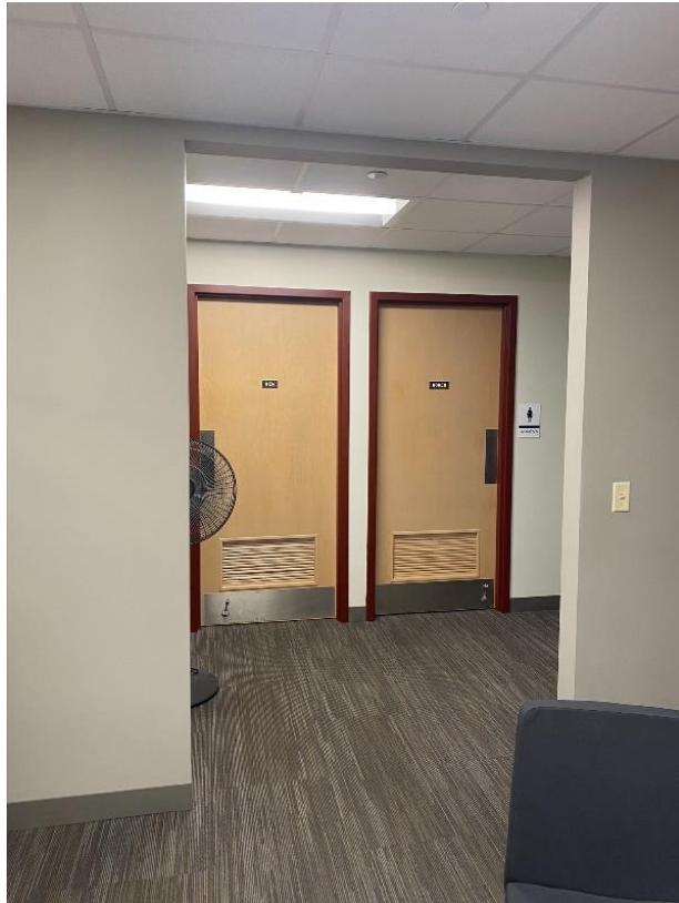
**Description:** Close in the current drywalled opening leading to the Assessor's restrooms allowing for extra privacy for staff and visitors. The project will entail filling in the open space with framing, installing a 36" solid core door, drywall and painting. This project is slated for the 2025-2026 fiscal year.
