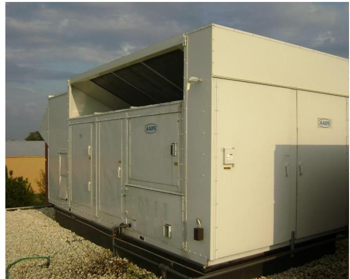
**Description:** The Community Center was constructed in 2006. The HVAC system for the addition involves two boilers, several pumps, and a roof top unit (RTU). All HVAC equipment is serviced on a quarterly basis in an effort to extend its useful life, however the RTU is aging and has a useful life of approximately 20 years. The RTU is targeted for replacement in fiscal year 2026-2027.
